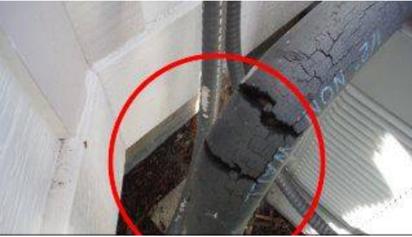
Photo 29-1 Insulation deteriorating
